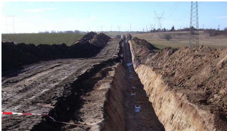
Figure 1 Typical trench excavation and construction on farm lands
