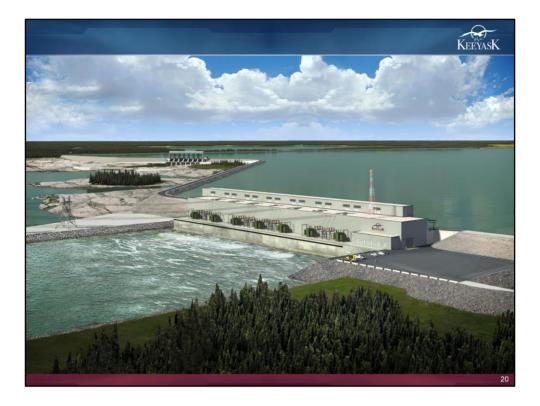
It will be a 695-megawatt hydroelectric generating station with seven turbines plus supporting infrastructure located at Gull (Keeyask) Rapids on the lower Nelson River 180 kilometres northeast of Thompson.
