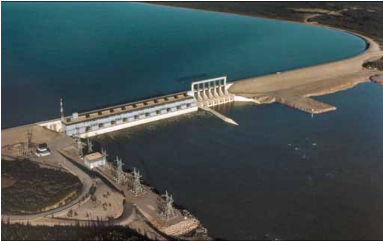
Long Spruce dam and generating station was the third plant built in the Split Lake resource area. Started in 1971, the first units went into service in 1977. It is located 16 kilometres downstream of Kettle.
