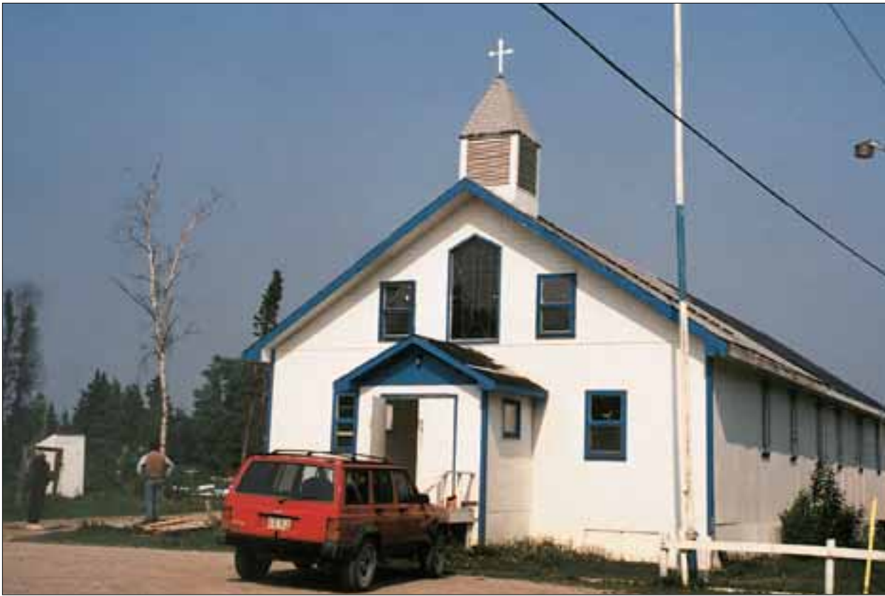
John the Baptist Anglican Church, built in the mid-1960s by Split Lake residents.
