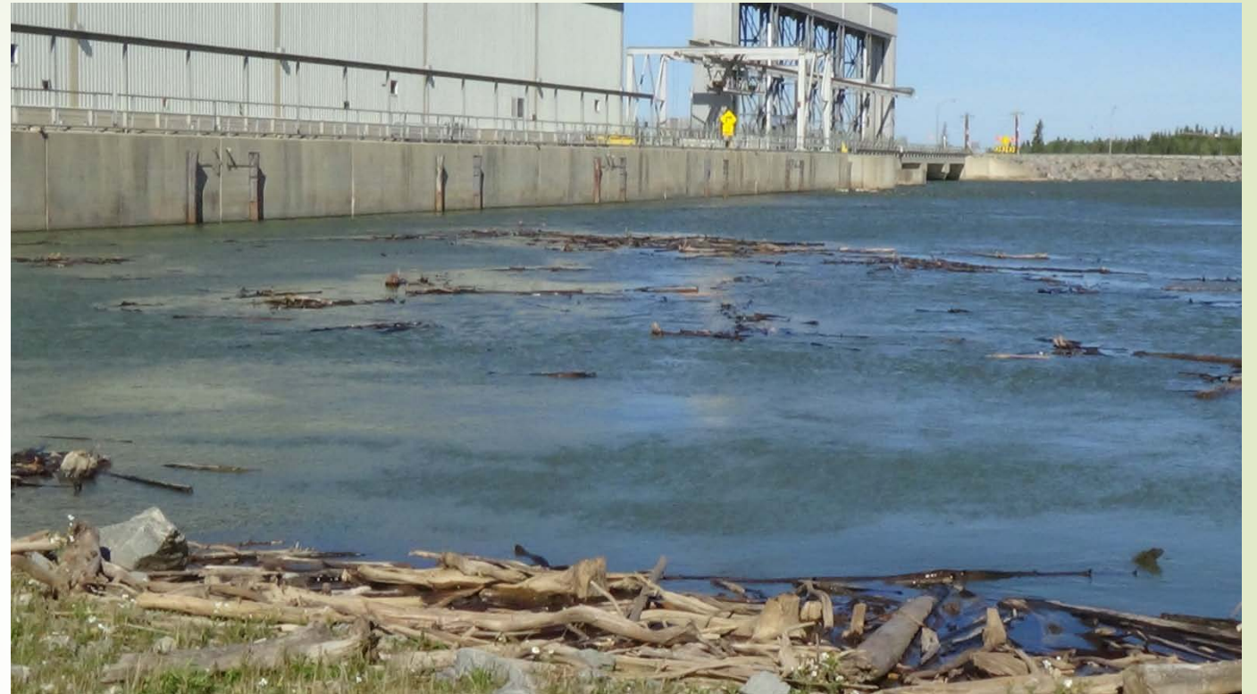
Jenpeg Generating Station Nelson River
