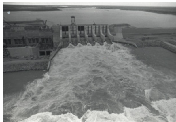
Long Spruce Generating Station, 1975.
