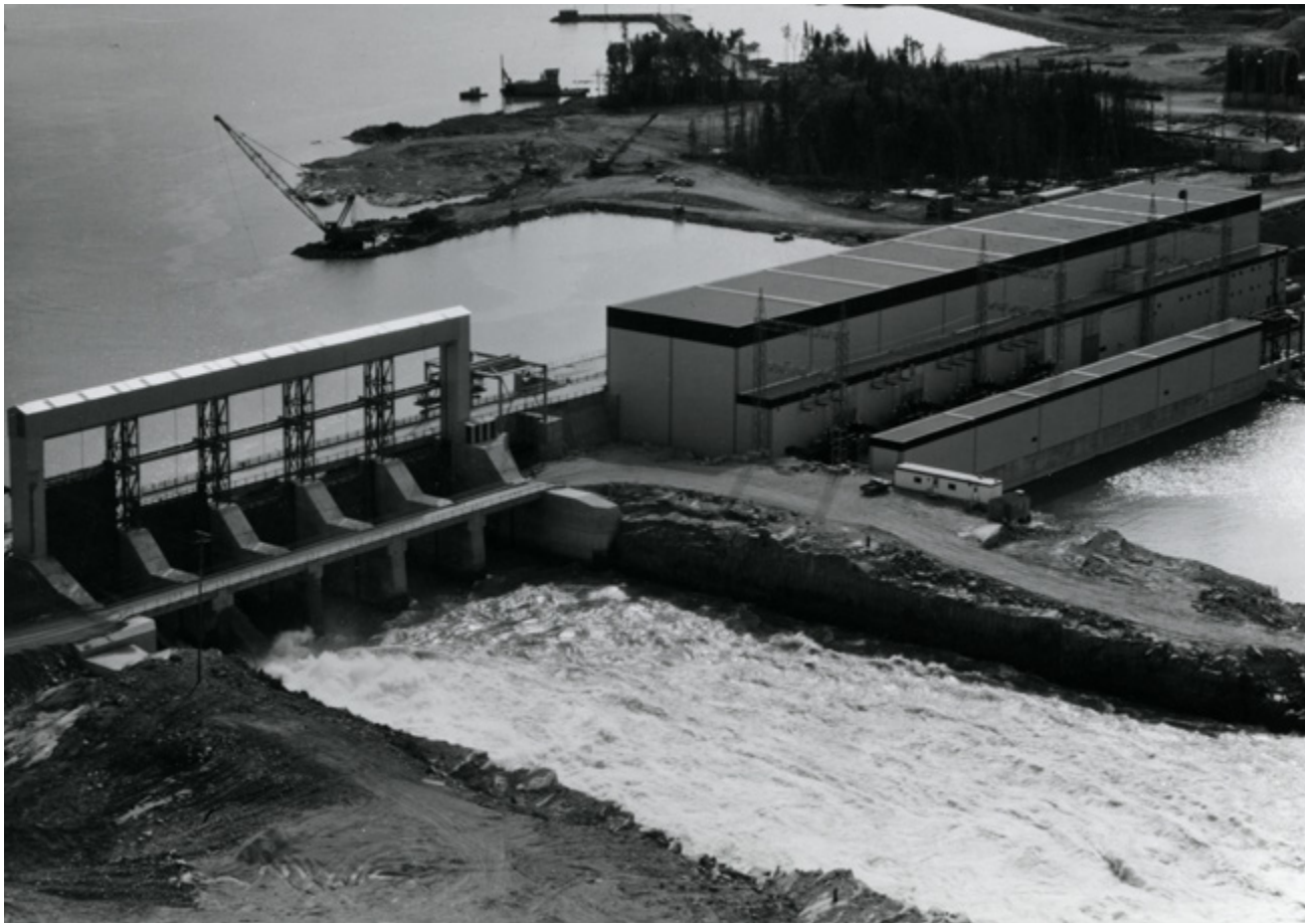
Jenpeg Generating Station, 1979.
