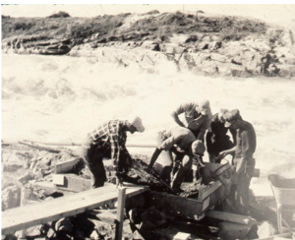
Construction of the Kelsey Generating Station on the Nelson River, circa 1958.
