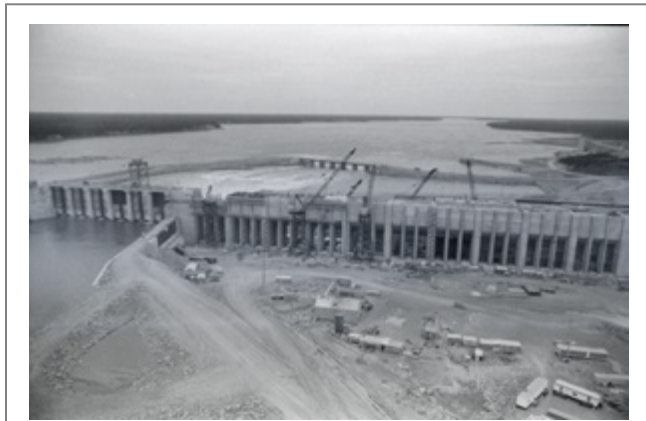
Construction of the Long Spruce Generating Station, 1975.
