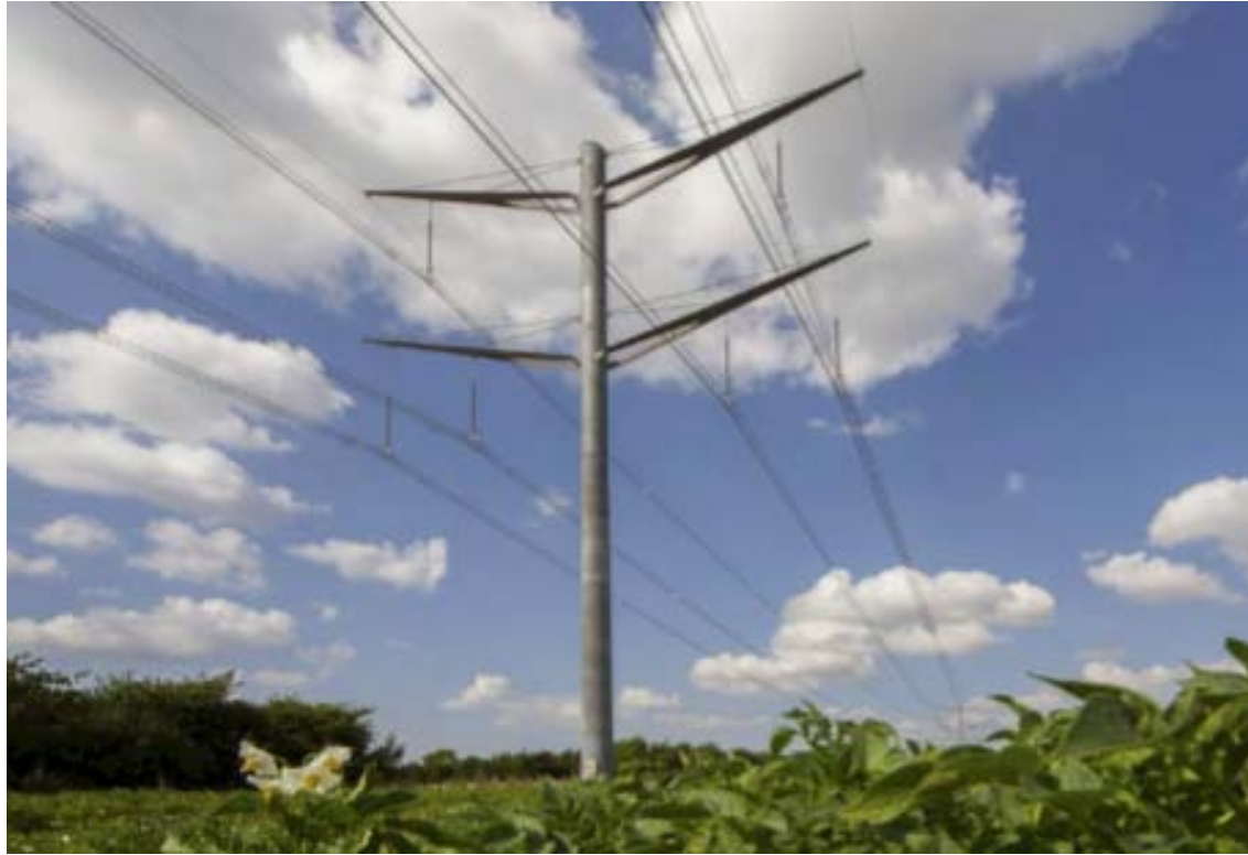
Figure 4 – New Tubular tower in Denmark
