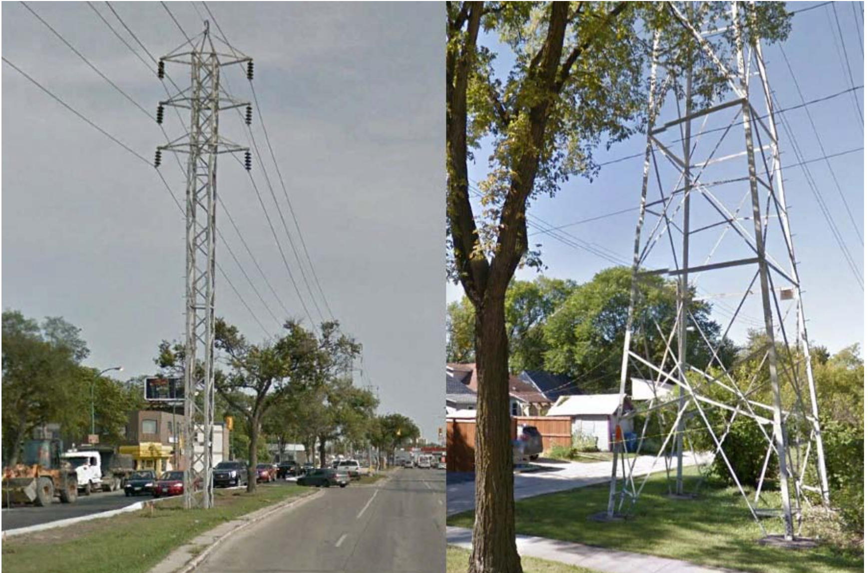
Figure 25 – Avoid property damage
