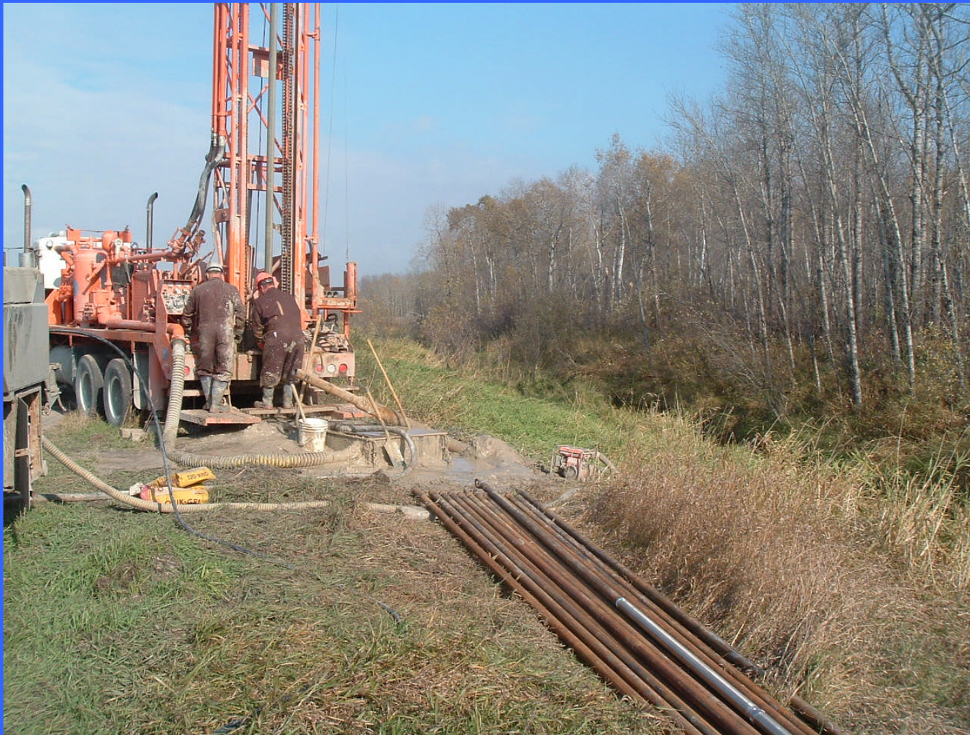
Testhole drilling to establish the geological setting
