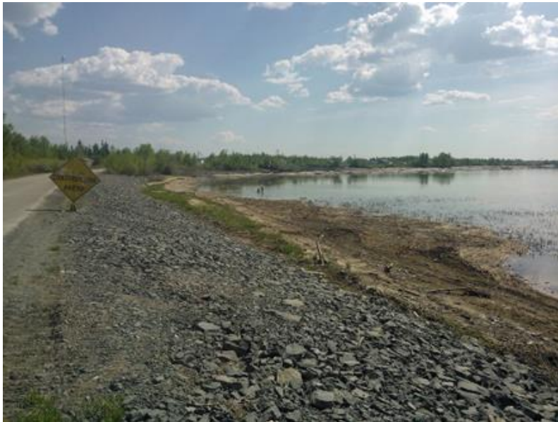
Armouring of shorelines to protect road bed and shoreline from high water. How much shoreline habitat has been degraded throughout the region due to threats of erosion?
