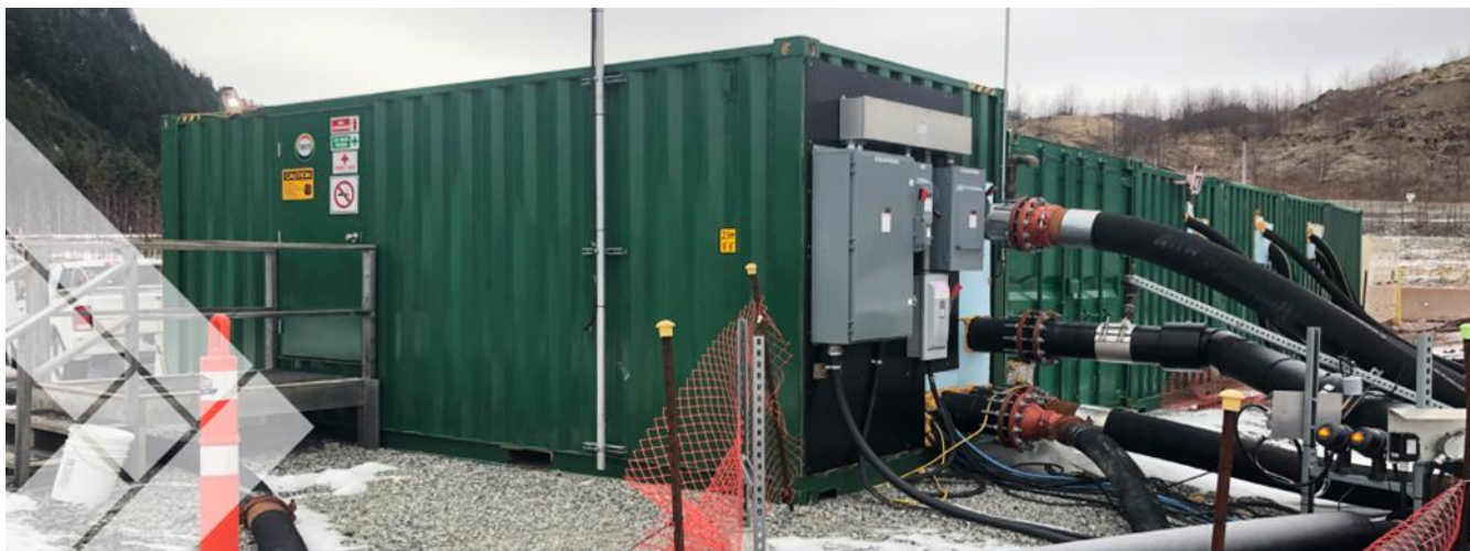
Figure 4-5: Chitosan Enhanced Sand Filtration (CESF) Management Systems (Figure Courtesy of SECURE)
