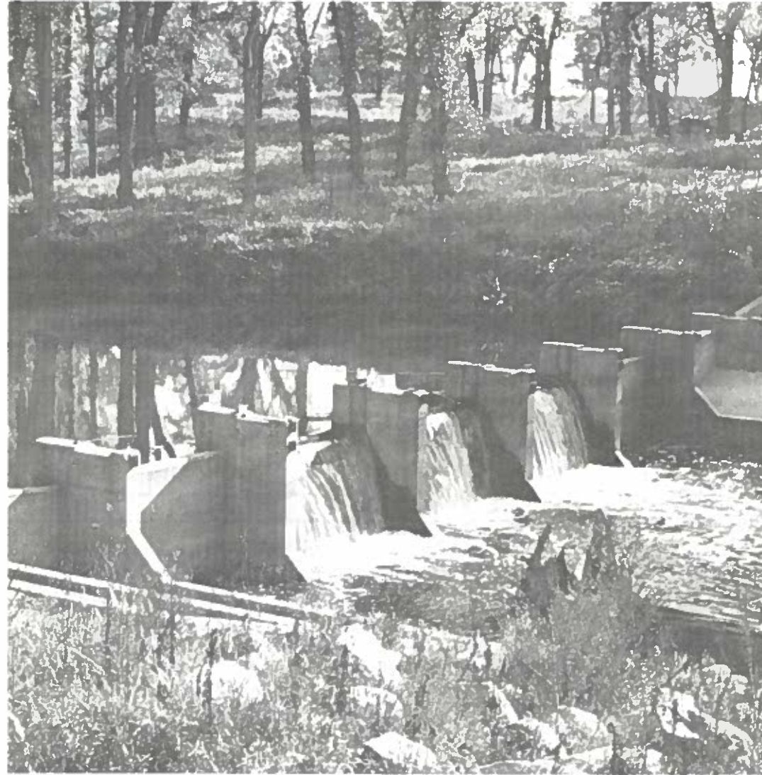
Dam, Roseau River at Dominion City
